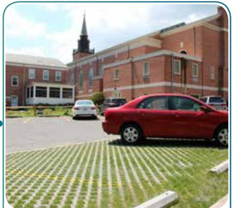
**Type:** Asphalt replacement and bioretention
